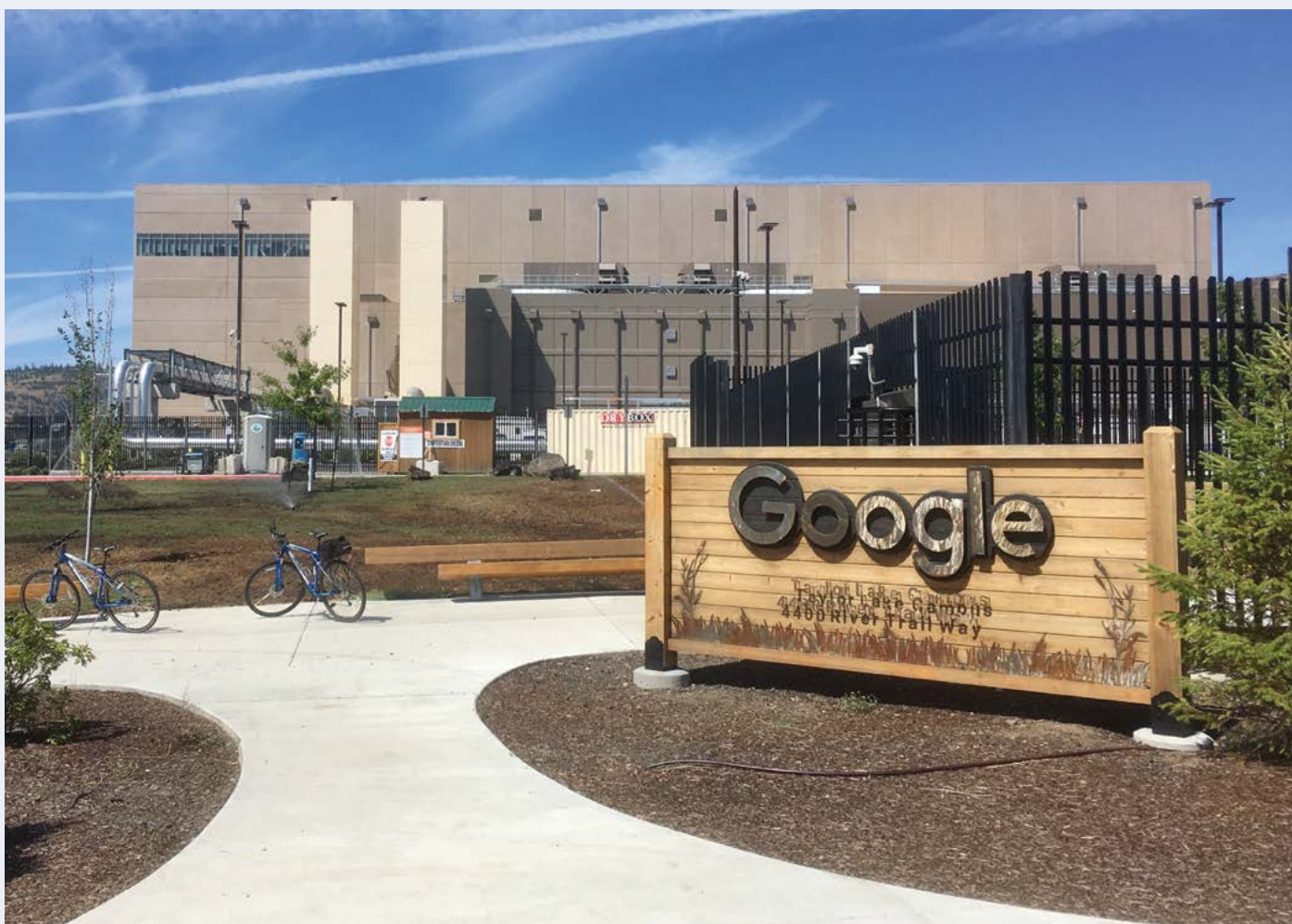
Google Data Centre. Photo Credit: Wikimedia
